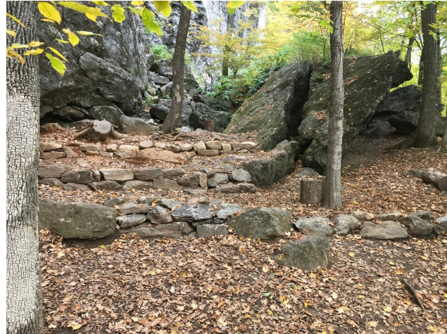
The left side of Meadows was extremely eroded. The CTeam built a series of retaining walls to stop future soil loss.
